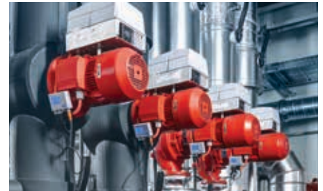
Etaline PumpDrive employed as dual-pump sets
