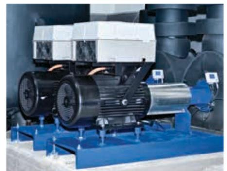
2 Etanorm PumpDrive pumps for continuous operation with high-efficiency KSB SuPremE® IE5 motors\*
